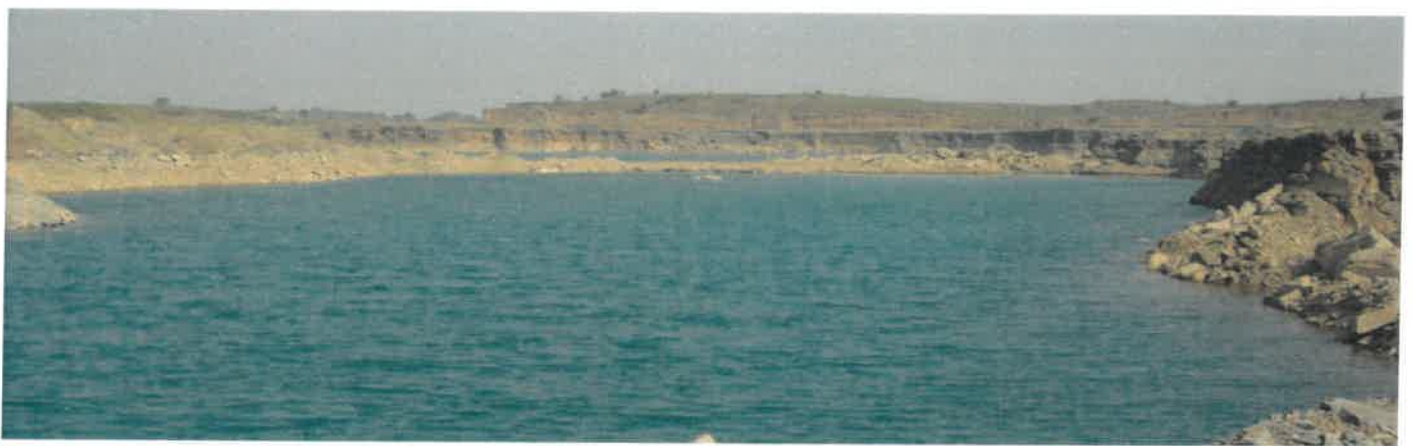
Water Reservoir in Narsingarh
